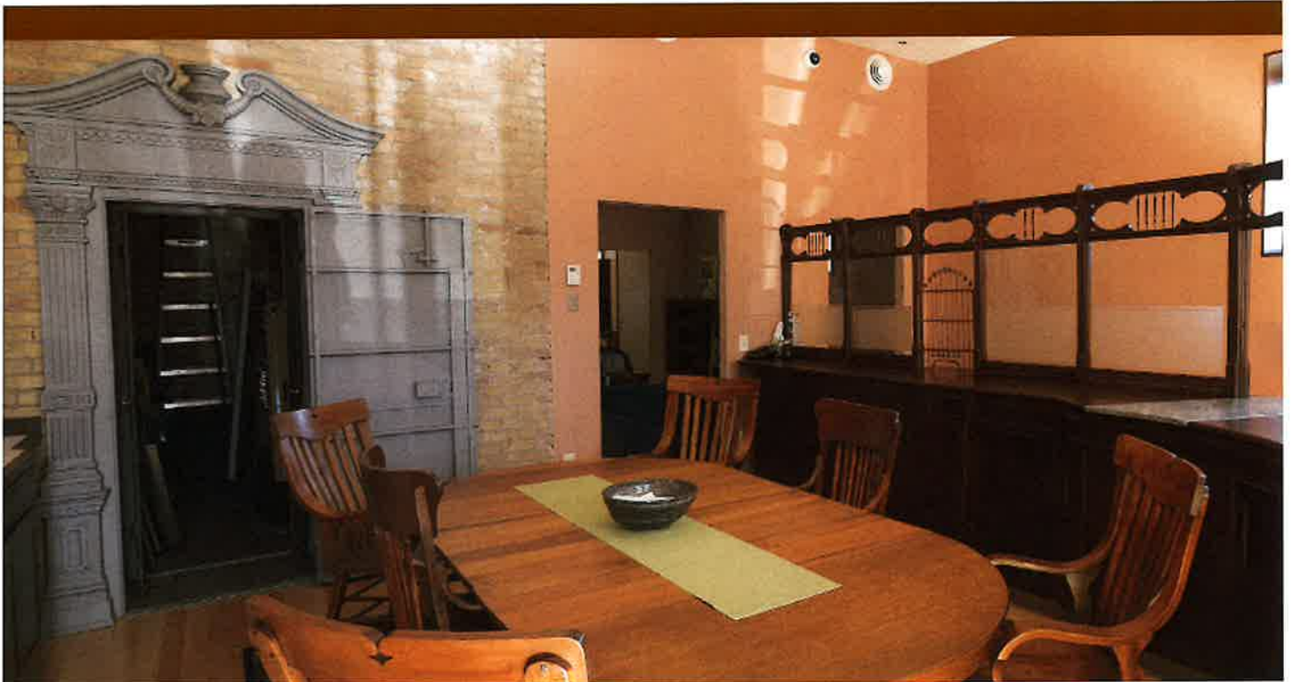
Photo illustrating progress made on the interior renovation
